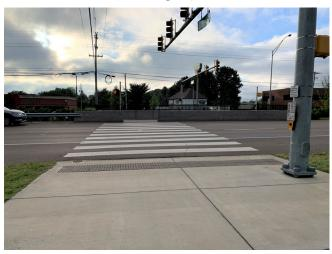
Figure 1: Signalized trail crossing with refuge. Source: FHWA
