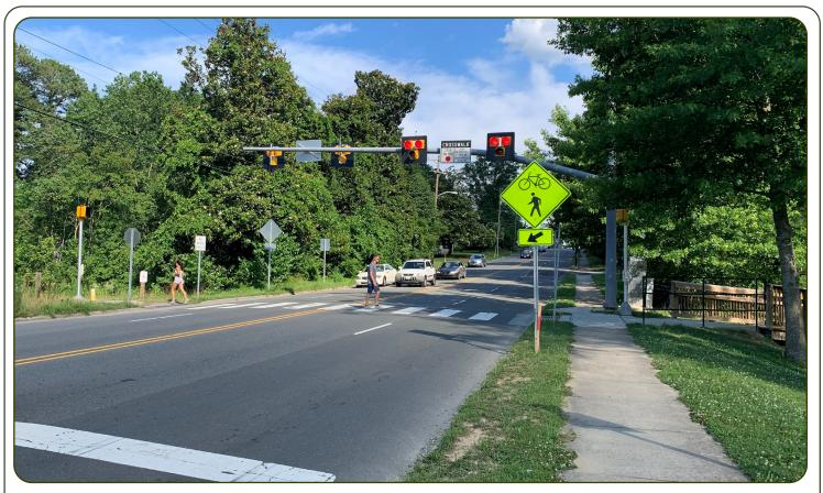
Figure 4: Mid-block trail crossing with PHB. Source: FHWA
