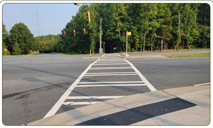
Figure 10: Trail crossing at a complex intersection with a wide refuge. Source: FHWA
