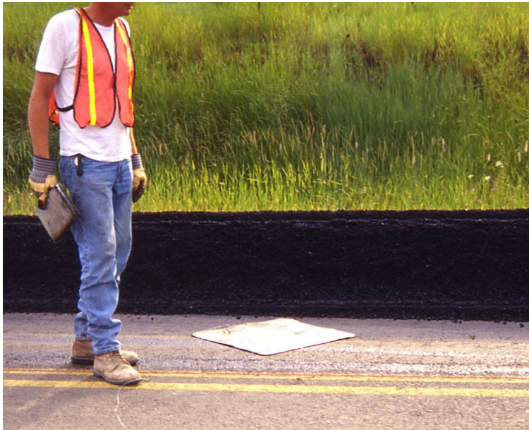
Exhibit 4-28 Obtaining Mixture Sample Prior to Compaction
