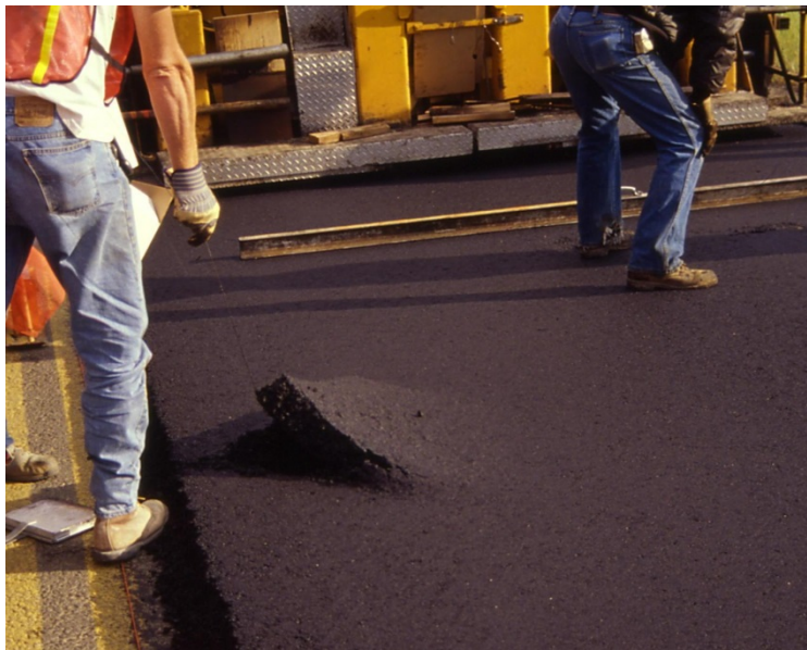
Exhibit 4-28 Obtaining Mixture Sample Prior to Compaction
